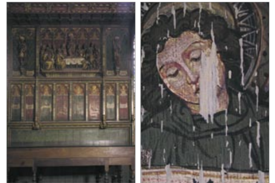
Figure 3 Details of the screen by G F Bodley at St Michael's Church, Cambridge, showing widespread and even delamination caused by adverse micro- climatic conditions
