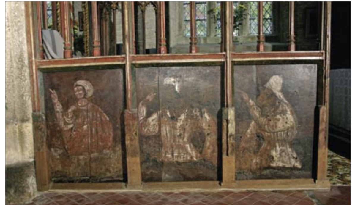
Figure 2 The screen at St Thomas Becket, Bridford, Somerset, showing patterns of deterioration at the base associated with historic capillary rise of ground water
