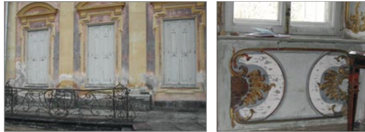
Figures 1a , b, c & d Deterioration of the painted panelling at the Chinese Palace, Oranienbaum, Russia, as a result of localised water penetration from the damaged terrace
